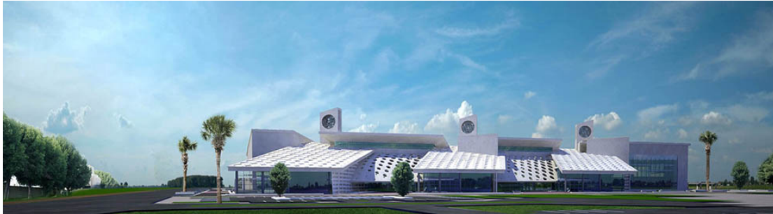
Figure I.2.2.1 College of Engineering newly operated building at H07 (source: CENG website)
